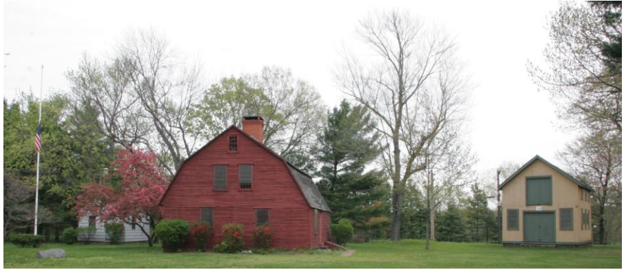
The 3 historic houses at Martin Park are, left to right, the 1820s Goodwin Schoolhouse, the 1761 Bemont (Huguenot) House, and the 1850s Burnham Blacksmith Shop.
